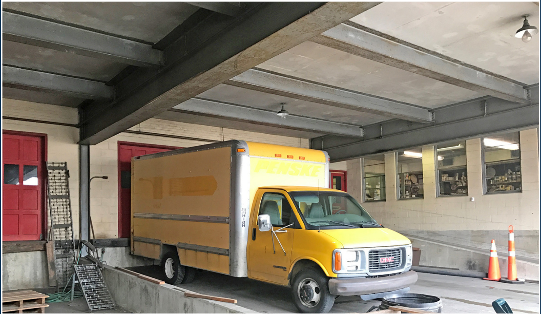
Two Interior Docks at 3'
